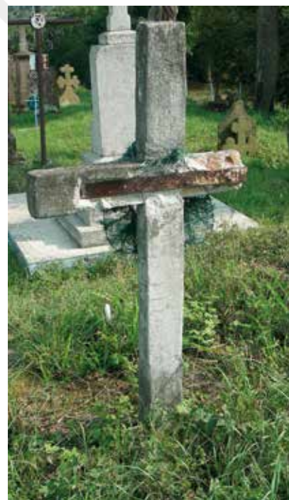
ILL. 38 Tombstone armature made of concrete (reinforced concrete)
