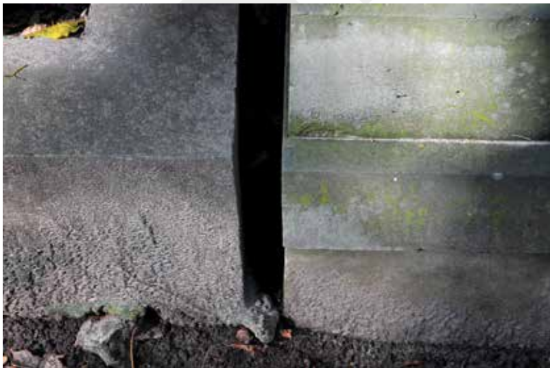
ILL. 55a Clearly distinguishable tombstone made of concrete (left) and one made of sandstone
