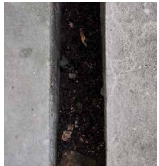
ILL. 55b Tombstones made of sandstone (left) and concrete (right) with a very similar texture making it difficult to distinguish the material
