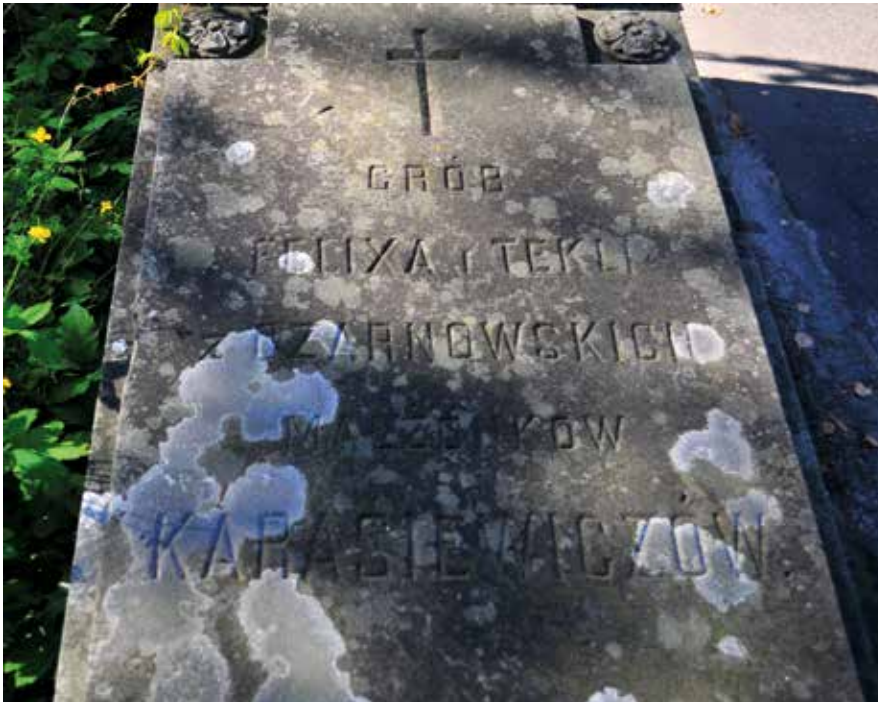
ILL. 57 Tombstone (made of sandstone) deteriorating due to weathering and lichens
