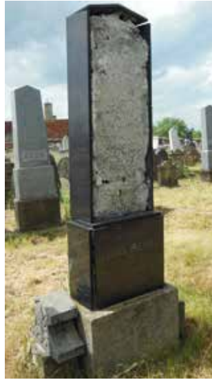
ILL. 40 Concrete tombstone (obelisk on a two-stepped pedestal) faced with stone slabs
